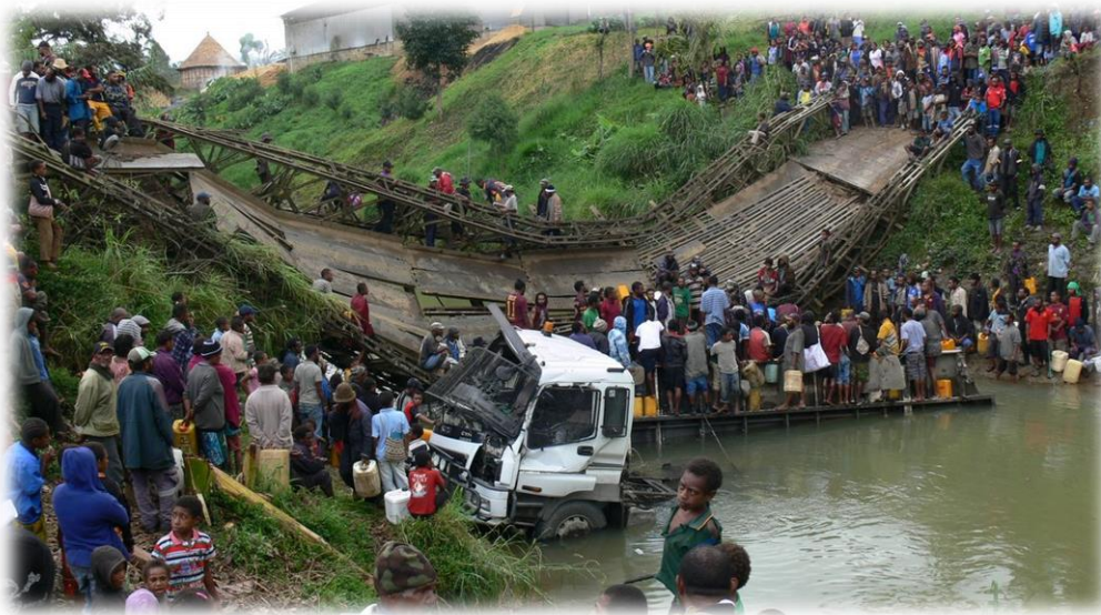
Collapsed bridge in Kainantu. 2014. What happened to the maintenance funds? http://www.thepostsinpng.com/2014/08/photo-journal-bridge-collapse/
