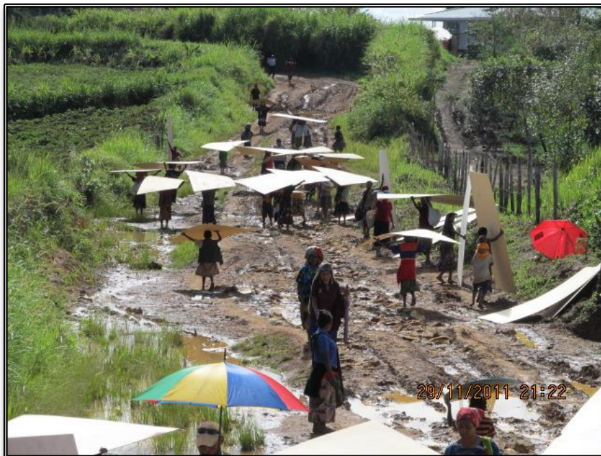
Taxpayers from a village carrying materials to build a clinic because of an impassable road in Western Province.
